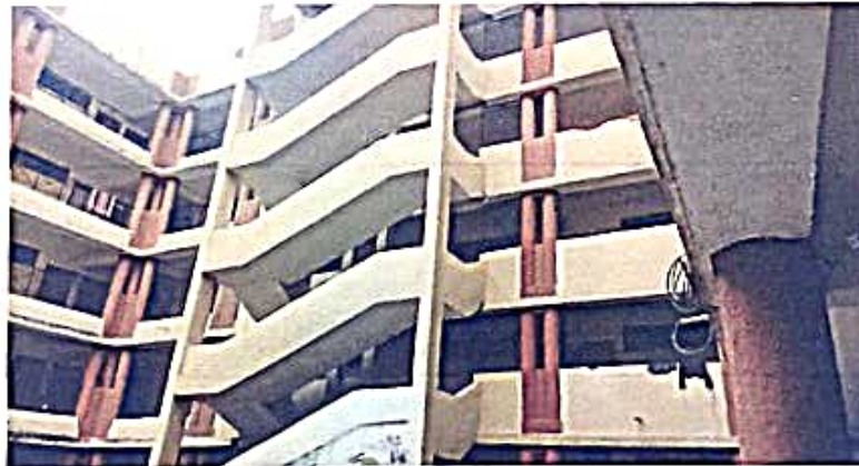
Photo: CCTV facilities in the entrance of Ladies Hostel
